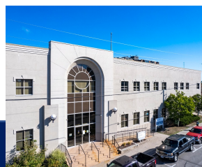
78 Richmond Street West 57,246 SF
